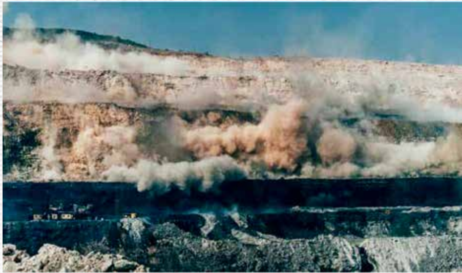
Figure 3: Coal mines blasting site [CMPDI brochure 2023]
